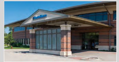
NorthShore's Ambulatory Care Center in Gurnee provides increased access for patients and families in Lake County.
